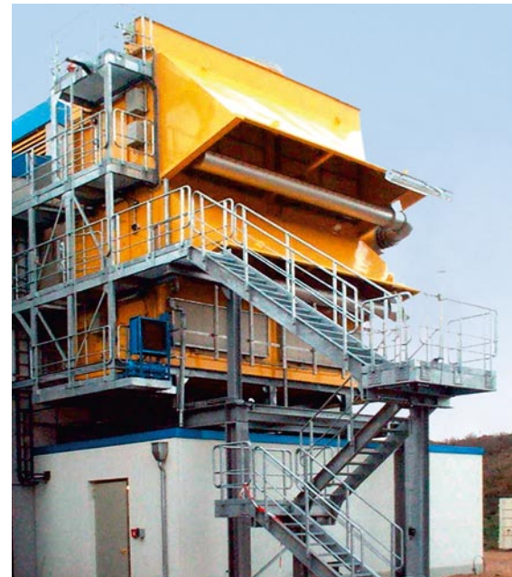
Static filter system with anti-icing
